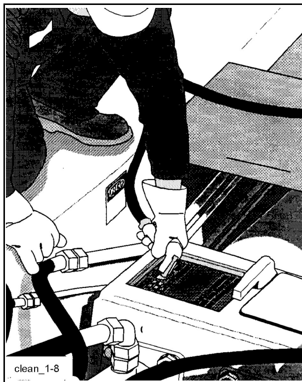
Fig. 130 Hose out water box
