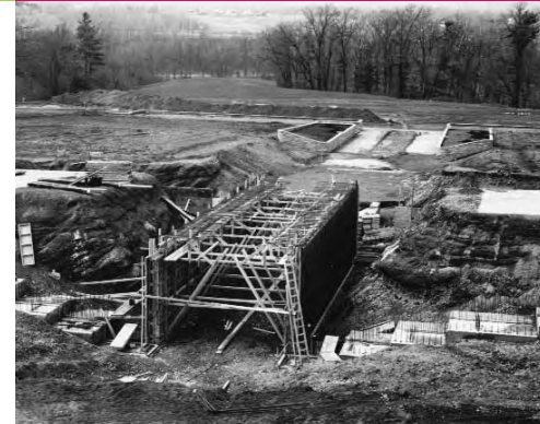
Underpass construction, 1964, and the beginning of Hendrie Park Gardens.
