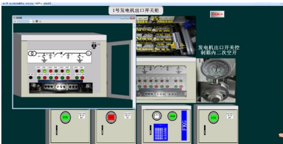
(a) Generator outlet switch cabinet switch operation
