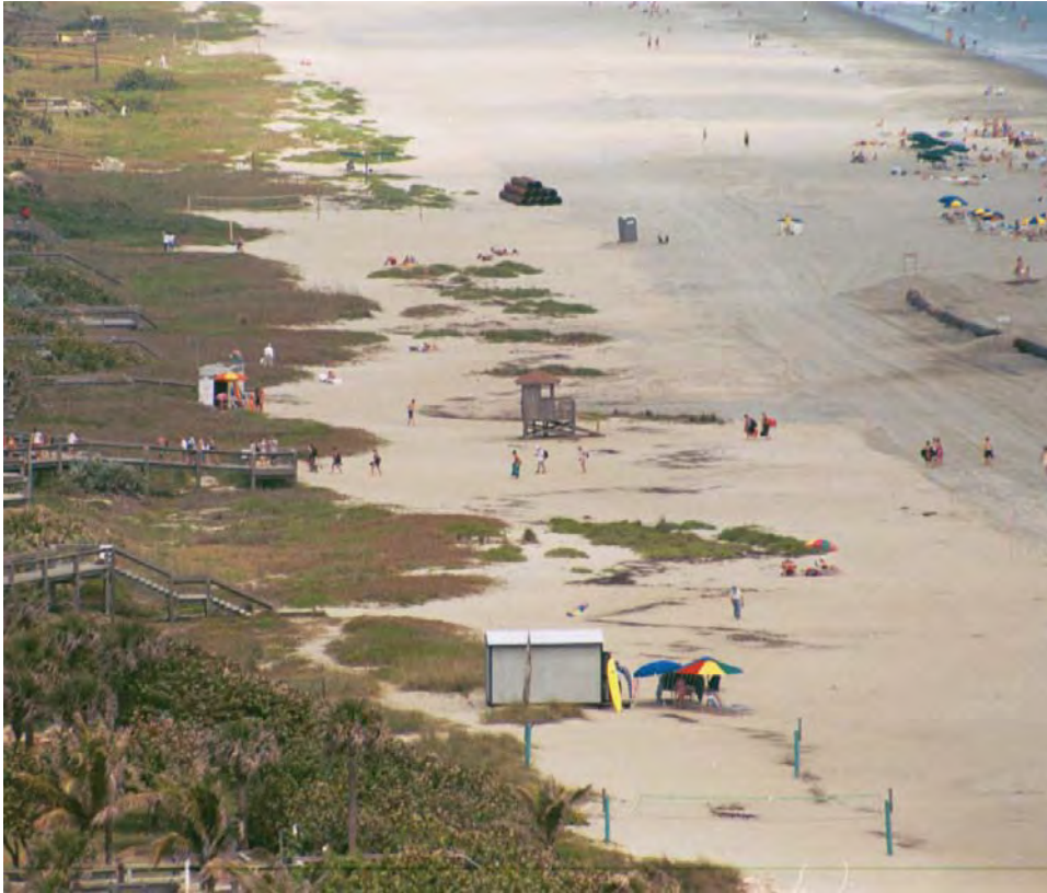
Figure 7-2: Beach fill material from Canaveral Shoals II borrow area (toward right of photograph) placed upon native Brevard County beach (toward left), several days after initial, hydraulic construction in 2001. (Brevard County Shore Protection Project, North Reach.)
