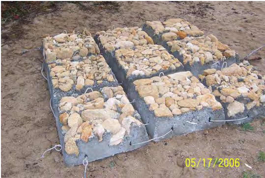
Figure 6-5. Articulated Concrete Mattress
