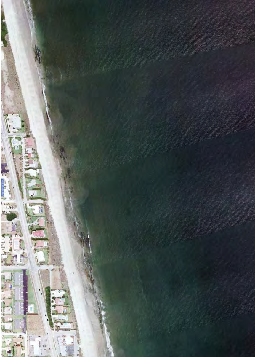
Figure 2-10. Aerial photograph of Mid-Reach exhibiting outcrops of exposed nearshore rock in June 2004 (vicinity of R-94 to R-97 within Reach 4).
