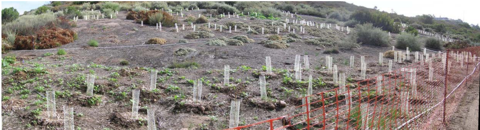
Post-installation, 09/01/11 Photo Location 10; Native grassland restoration.
