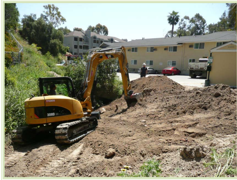
1830 Upas Street Sewer Pipeline Repair
