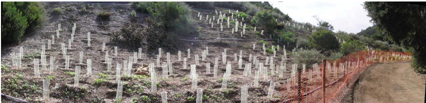
Post-installation, 09/01/11 Photo Location 11; Native grassland restoration.
