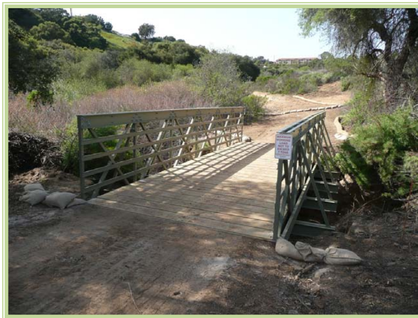
Tecolote Canyon- New Access Bridge
