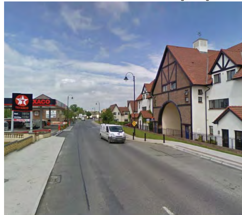
Photo 3.6: Pedestrian Barrier & Absence of Crossings along Main St.
