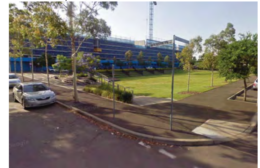
Photo 7.6 Example of Water Retention Park
