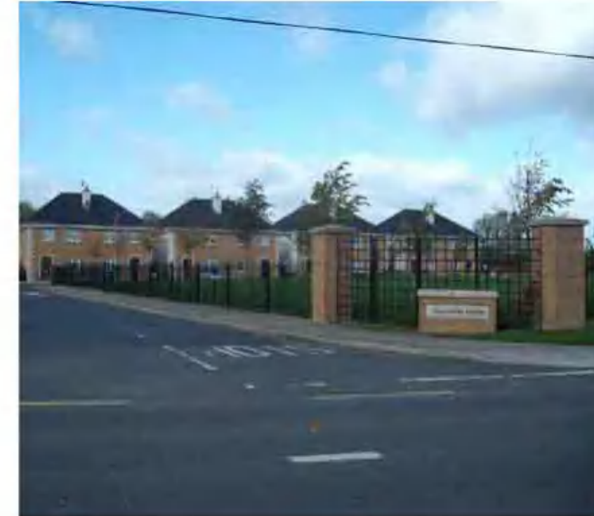
Photo 3.8: Enclosure of Public Open Space with Pedestrian Guardrails
