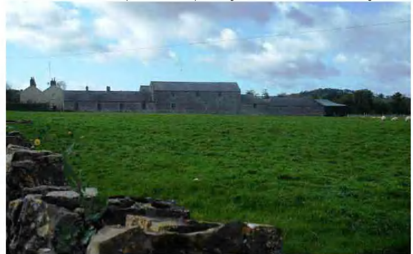
Photo A2 View of Newcastle Farm (Protected Structure) Across Agricultural Lands at Western End of Village
