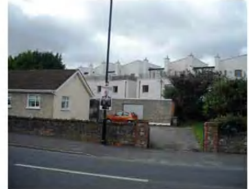
Photo 3.3 Urban & Rural Type Development on Eastern Side of Village
