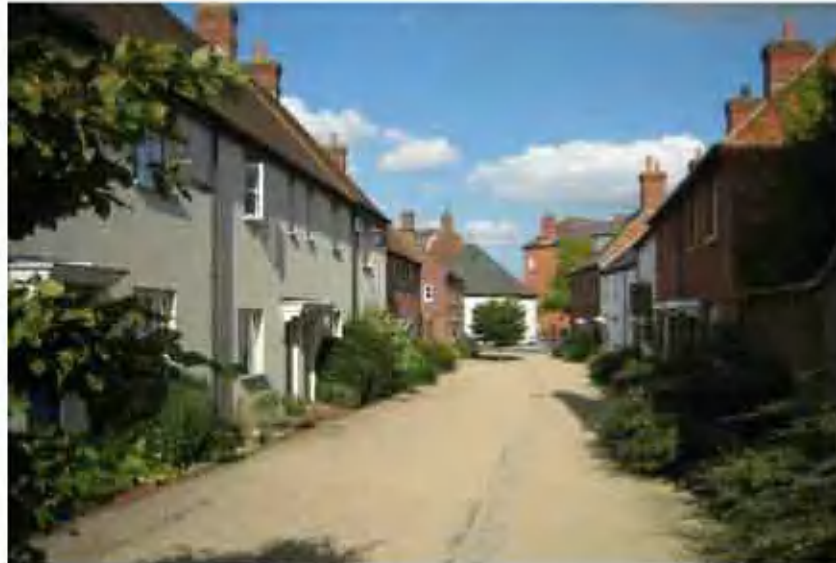
Photo 7.1 Example of Shared Surface Street
