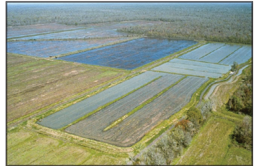
Baffle levees for water circulation
