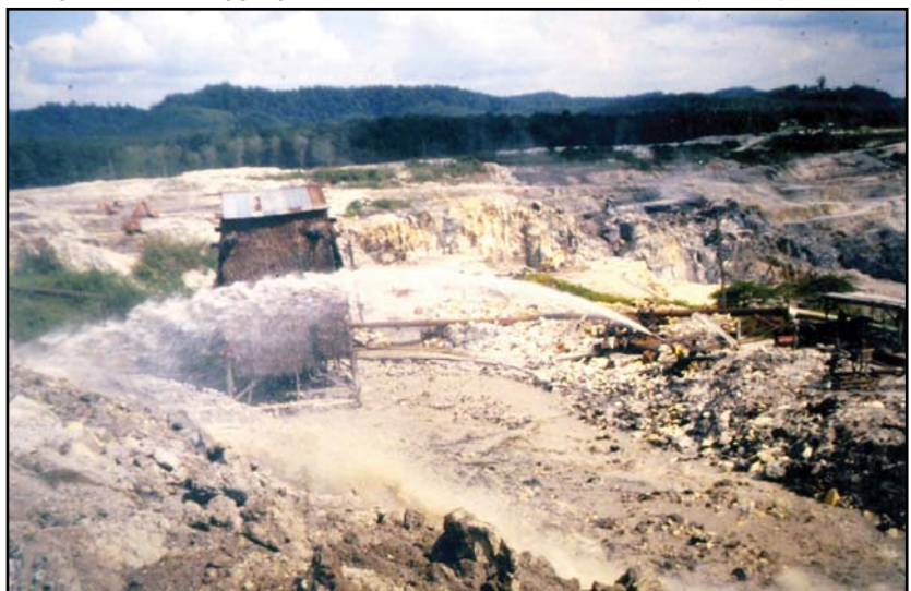
Below, 3: Hydraulic tin working with monitor (water) & limestone “pinnacles” being worked for aggregates. Unitex Tin & Limestone Quarry, Malaysia.
