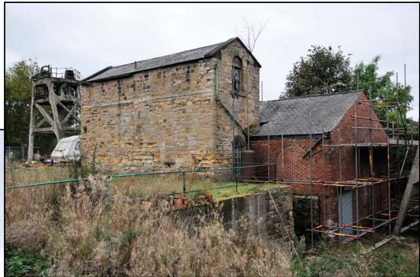
Right: The winding engine house at Hemingfield Colliery with the second concrete headframe at the far end of the building.
