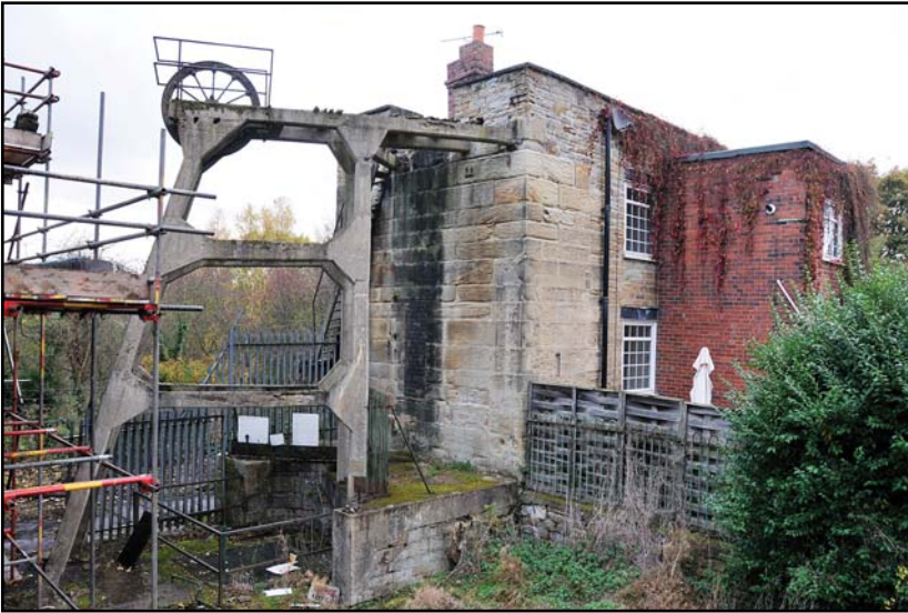
Right: The winding engine house at Hemingfield Colliery with the second concrete headframe at the far end of the building.
