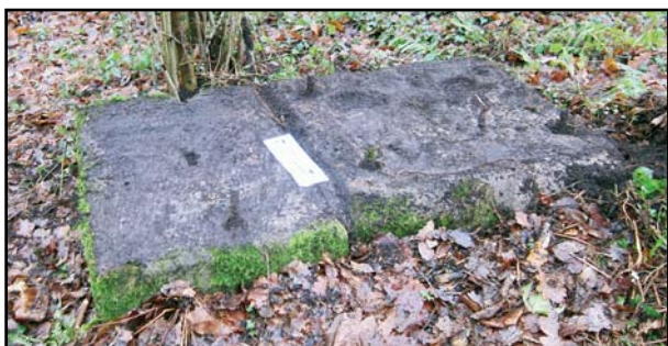
Engine bed for an upright (vertical) steam winding engine. SJ 68460 01895. (S.Dewhirst)
