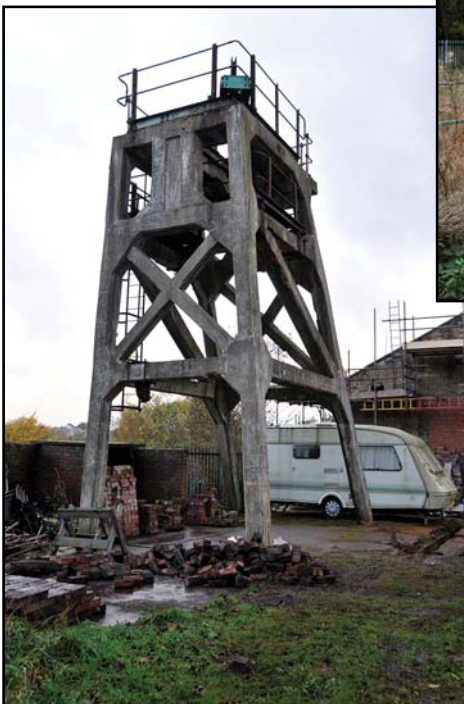
Left: One of the two concrete headframes at Hemingfield Colliery.
