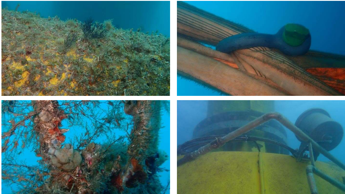
Figure 5 Different structures show different stages of fouling
