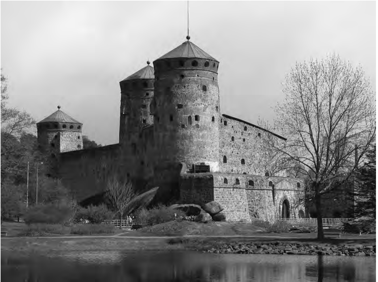
Fig. 4. Olavinlinna Castle from the west. The uppermost floors of the towers with round loopholes were laid with bricks in the 18th century. Photo by Terhi Mikkola / NBA, Olavinlinna Castle.
