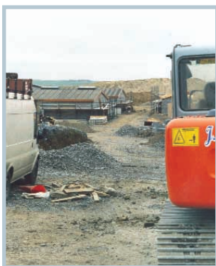
▲ New Nursing Home in Strandhill under construction
