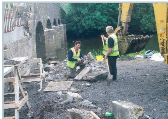
▲ Sligo County Council Staff working on the reconstruction of Templehouse Bridge
