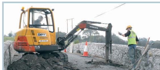
▲ Construction work on Lisconny Bridge
