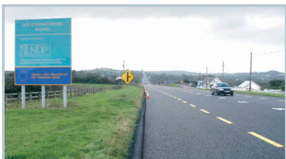
▲ N15 Strengthening Works
