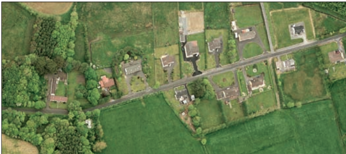
Ribbon development: frontage development along a road with no tandem development in the backlands
