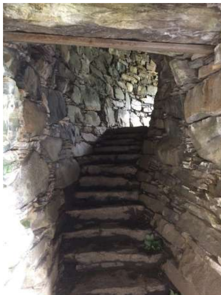
The distinctive double wall of a broch, balla nam fianntaichean , at Dun Telve, Glenelg. Photo © Meg Bateman
