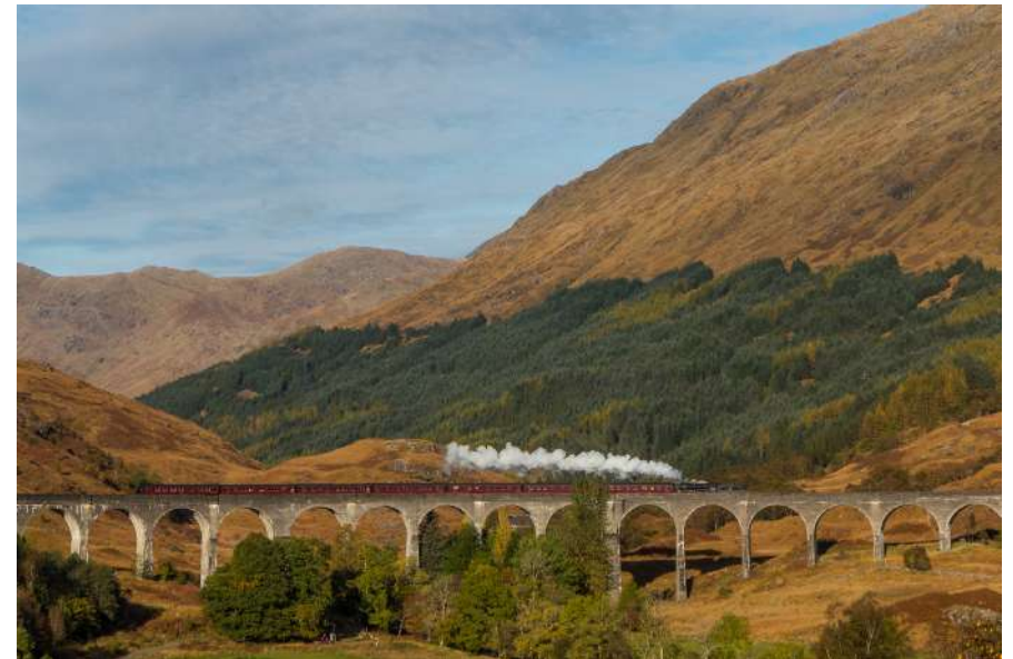
Glenfinnan Viaduct. Photo © Seán Purser
