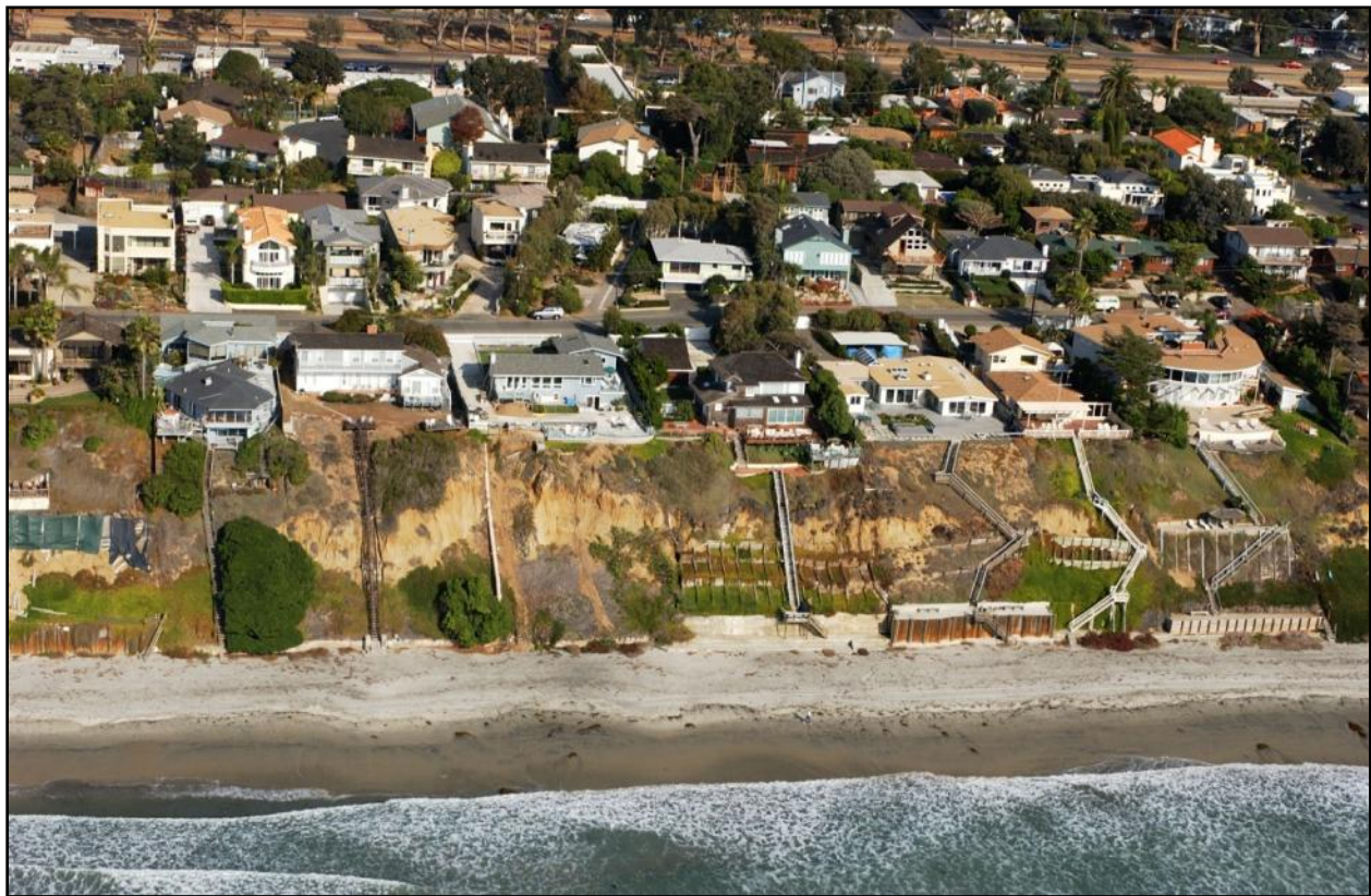
19 20 Figure 1.8-3 Portion of Reach 1
