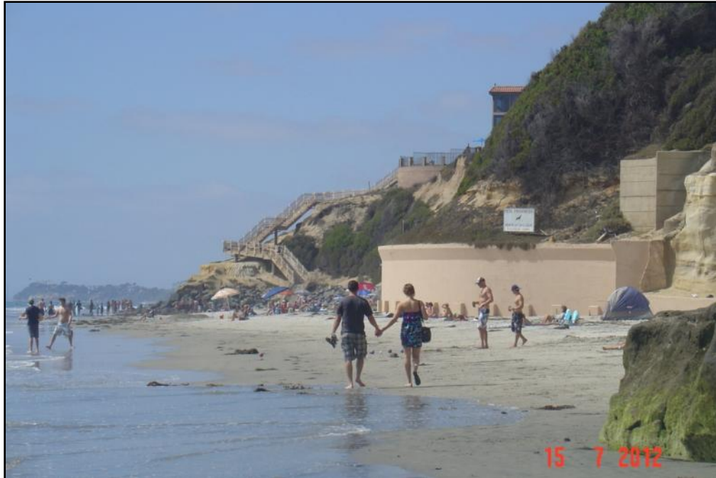
1 2 Figure 4.7-14 Solana Beach Receiver Site: from south end looking north
