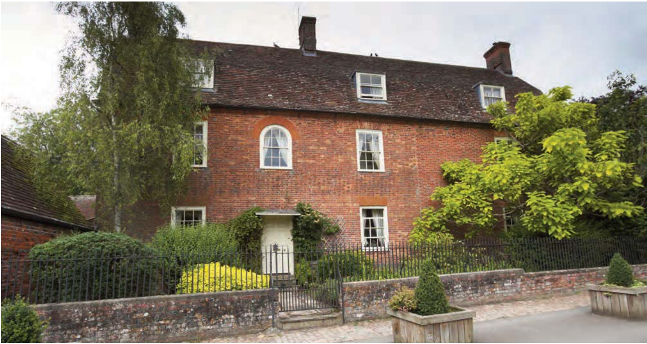
Plate 43 Iron railings on low stone brick walls, High Street, Avebury (© Erica Gittins)
