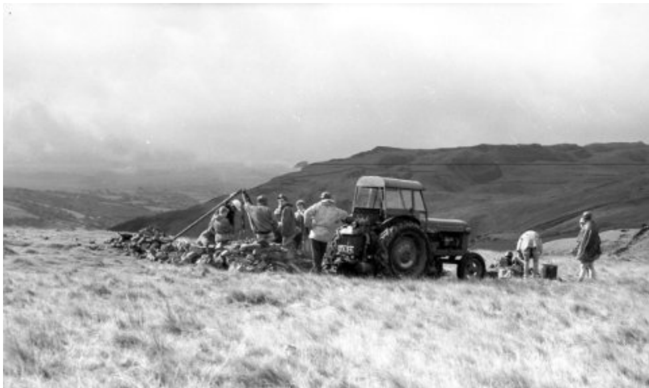
Digging Tunnel Cave Top Entrance. Note the Holman compressor mounted on the tractor. (©Dai Hunt, SWCC Archive: DHUNT_067)
