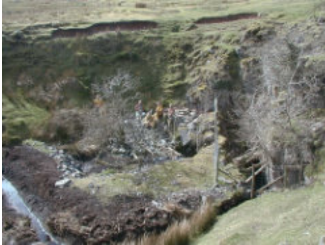
Digging Team on-site in 2007. Witness the very neat water-diversion works, bottom left.
