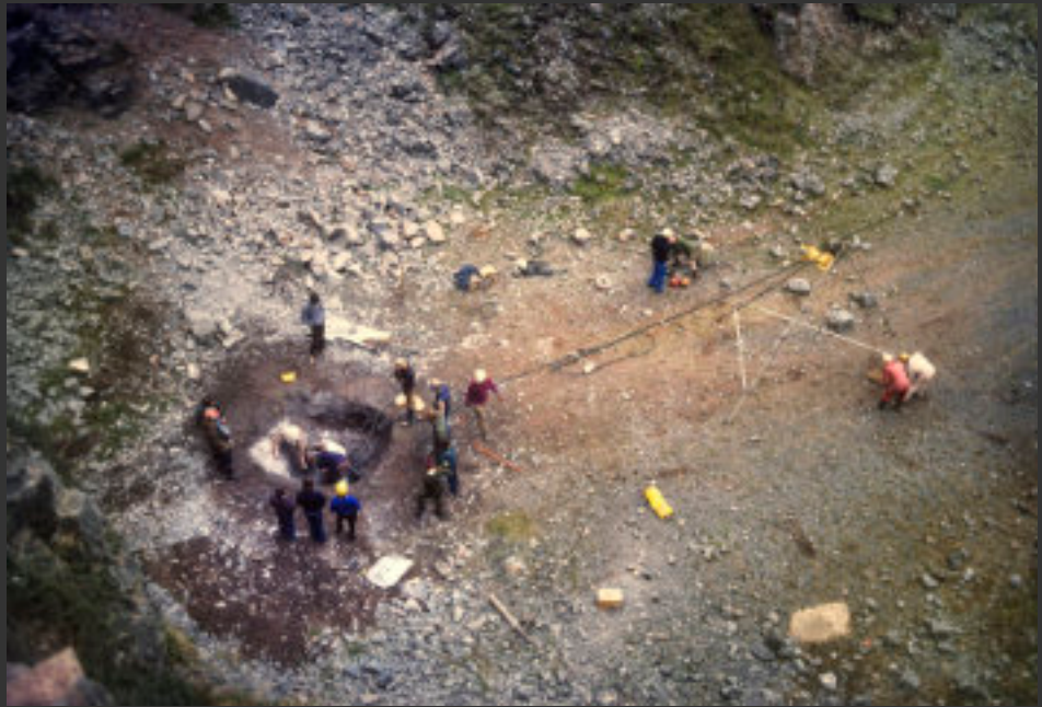
Work well underway after the first round had been cleared
