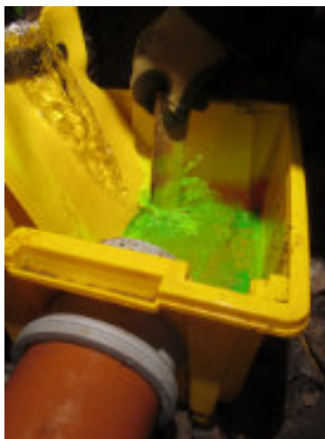
Fluorescein dye being mixed and added to the pipework system in Ogof Giedd, 5 th Jan 2020
