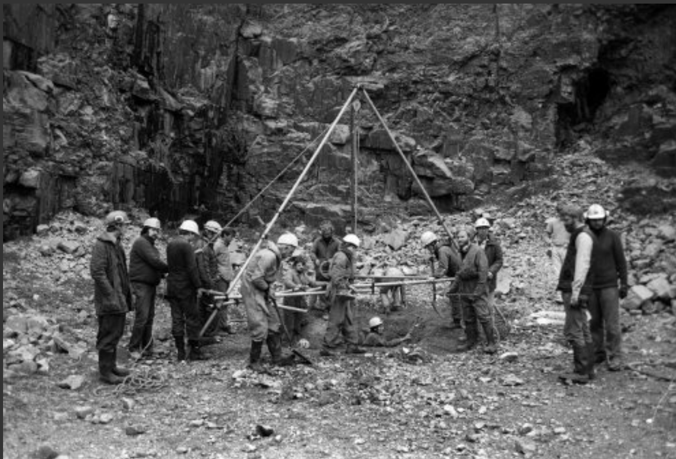
Below. The dig in action. The tripod was lifted and carried to one side before drilling and blasting.
