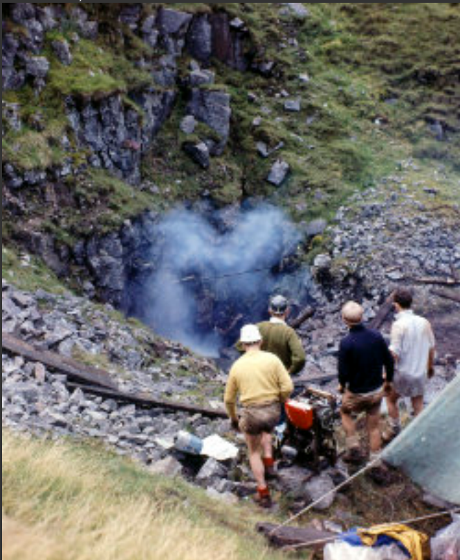
Work at the sink at Waun Fignen Felen in 1963 (©Dai Hunt)
