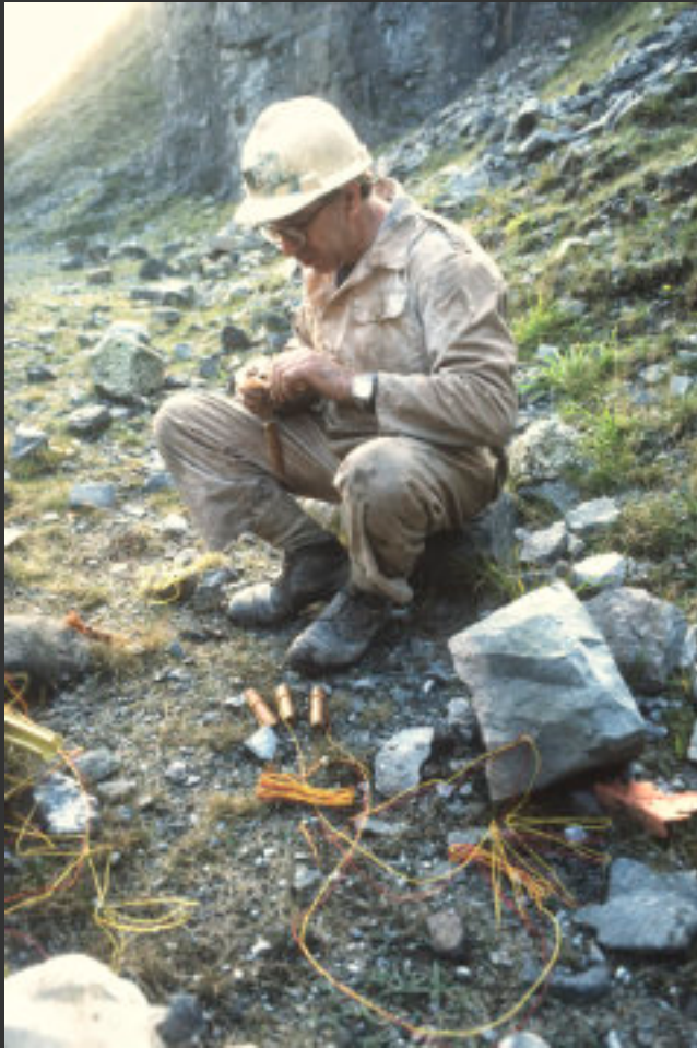
Roger, 'The Bomber', Bryan priming charges with delay detonators
