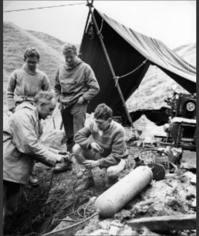
Waun Fignen Felen. Front L to R: Clive Jones, John Harvey. Others unknown. Diving cylinder for pneumatic chisel in foreground, generator back right (Photo probably by Glyn Genin)
