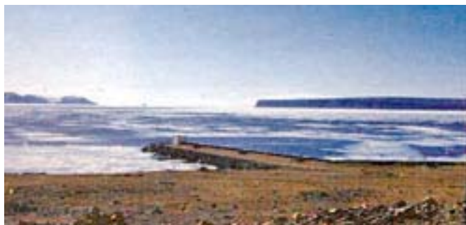
Thule Air Base Pier
