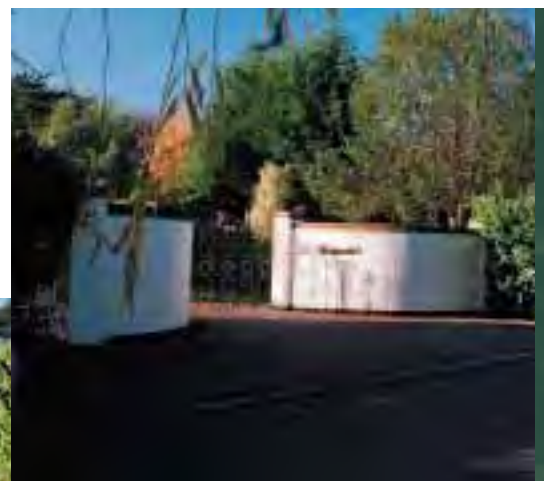
Gates and walls
