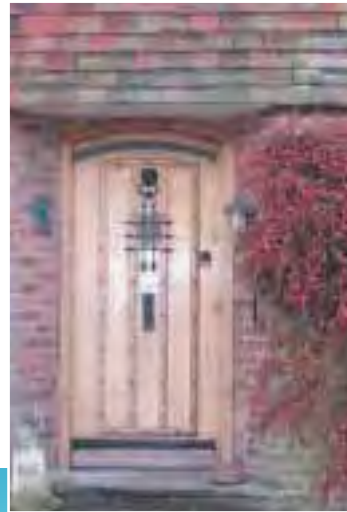
Front doors and porches
