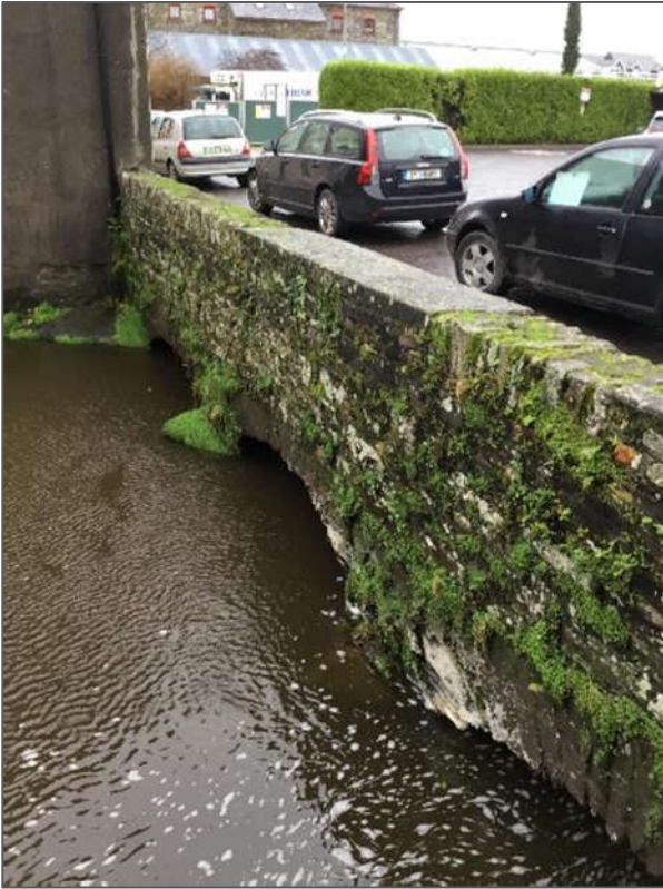
Plate 2-5 Clarke Street Bridge.
