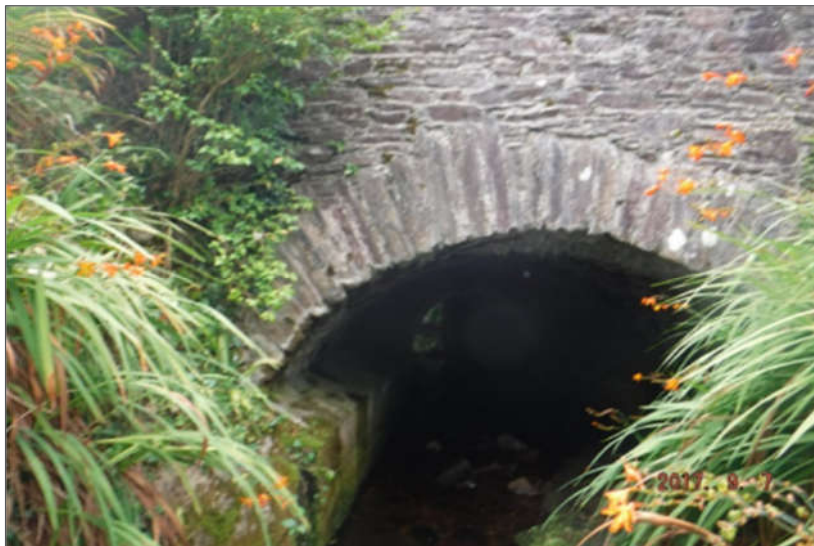
Plate 5-17 Kilnabrack Upper Bridge.
