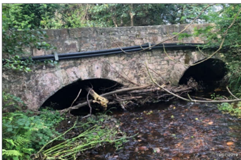
Plate 2-13 Kilfeighny North Bridge.
