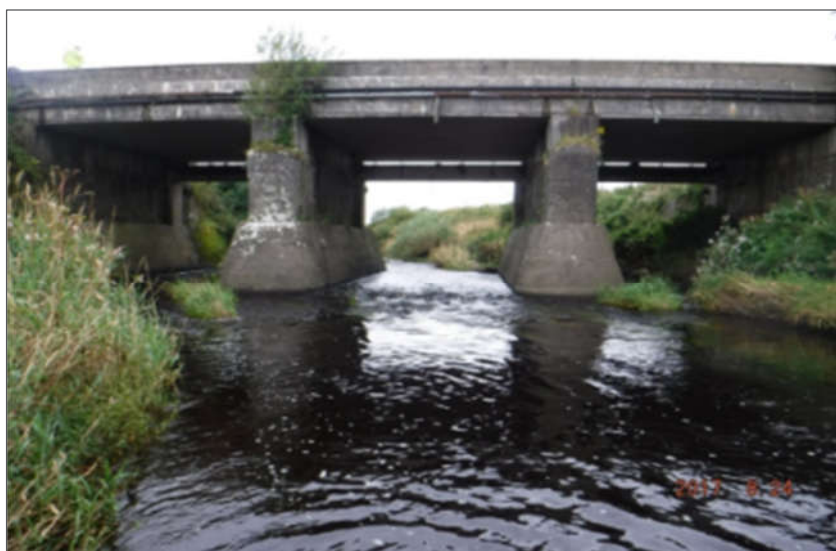
Plate 5-11 River Galey Bridge.
