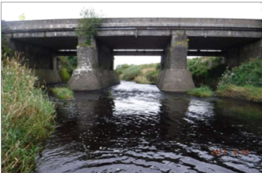
Plate 2-11 River Galey Bridge.
