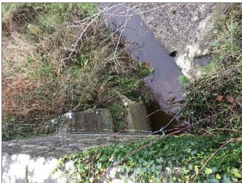
Plate 2-12 Galey Bridge Culvert.
