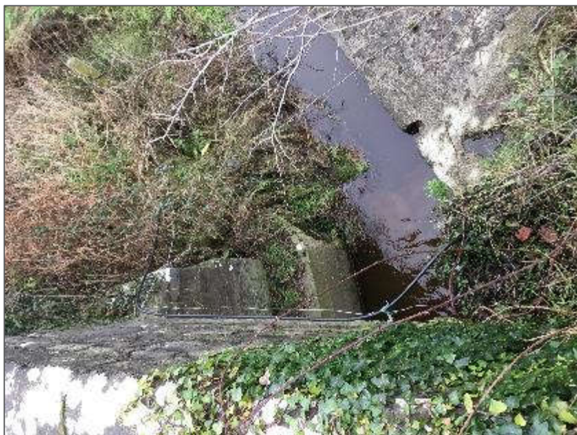
Plate 5-12 Galey Bridge Culvert.
