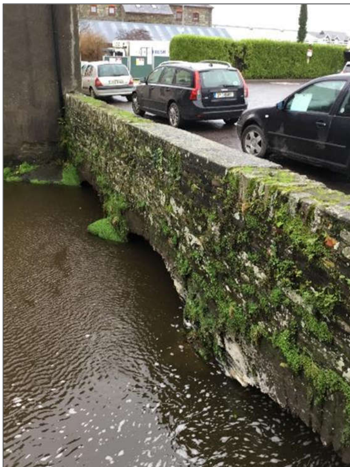
Plate 5-5 Clarke Street Bridge.
