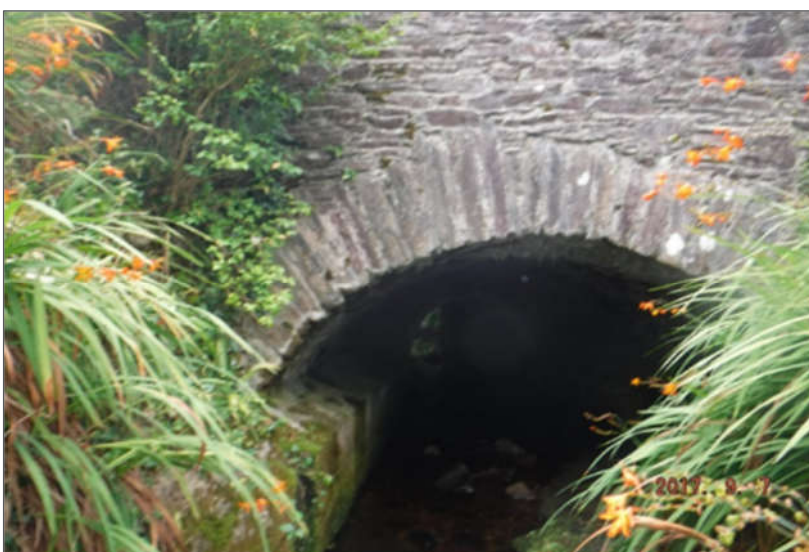
Plate 2-17 Kilnabrack Upper Bridge.
