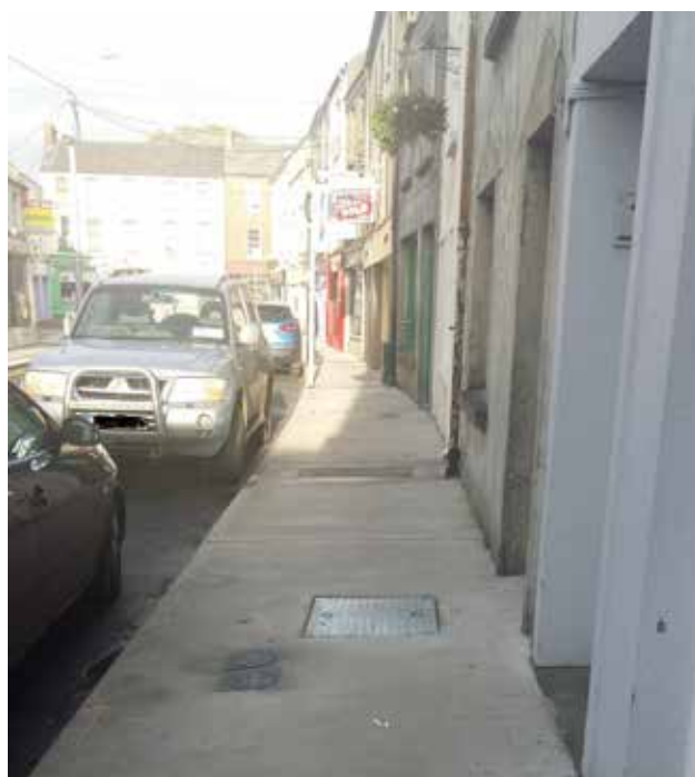
Footpath Improvements Croke Street
