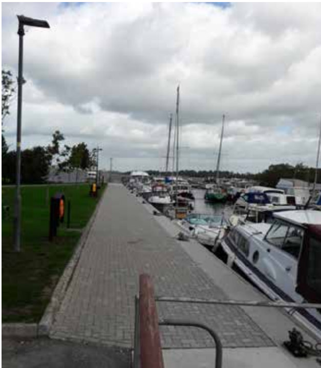
Town & Village Renewal 2017 Scheme funded Pier Refurbishment project in Terryglass
