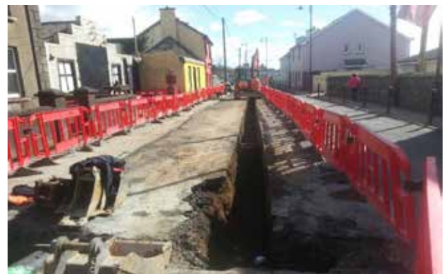
Ballina Watermain Rehabilitation
