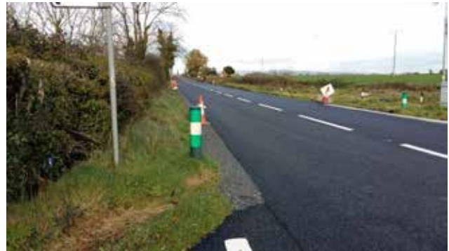
Works at Lismackin, Roscrea, November 2018
