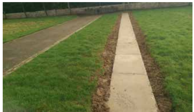
New plinth at grange burial ground
