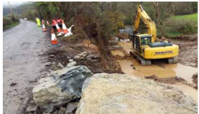
Road repair in progress by Clonmel Borough District following storms in 2018
