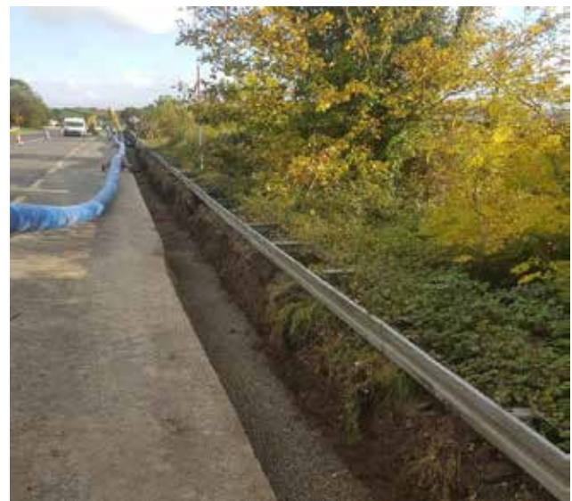
Fawnagowan, Tipperary Watermain Rehabilitation
