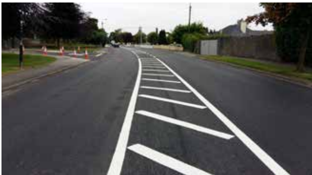
Works at Slievenamon Road, Thurles, June 2018
