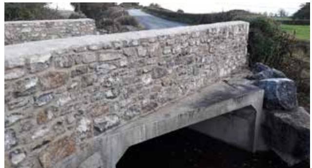
Bridge works completed in 2018, Moyglass, Carrick on Suir District
