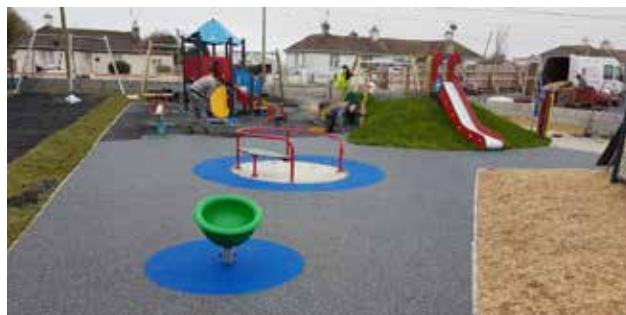
CLÁR Scheme funded playground under construction in Gortnahoe
