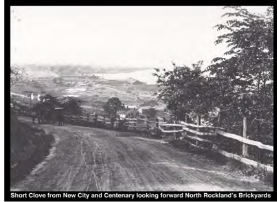
Short Clove from New City and Centenary looking forward North Rockland's Brickyards
