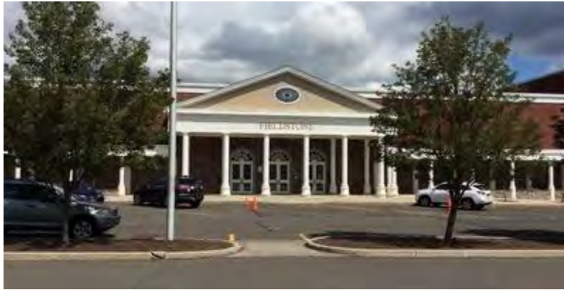
Front Entrance of Fieldstone Secondary School
