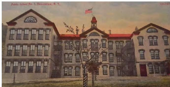
Haverstraw High School on Hudson Avenue
