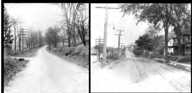
Road before 9W was completed. Probably road from West Haverstraw to Stony Point.
