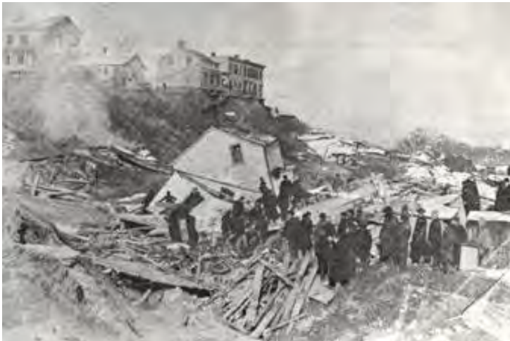
Photo showing the aftermath of the 1906 Landslide
