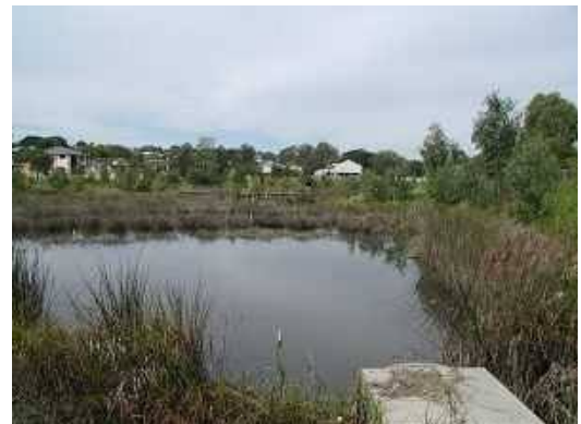
Plate 4-1: Example of Soft Edge Embankment Planting
