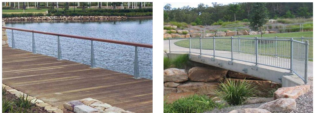
Plate 4-5: Typical examples of safety fencing to water edge
