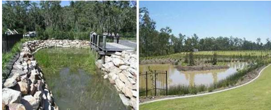
Plate 4-2: Examples of Hard edge Treatment for Open Waterbodies
