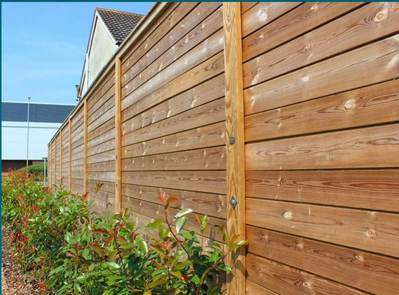
Timber acoustic barrier
