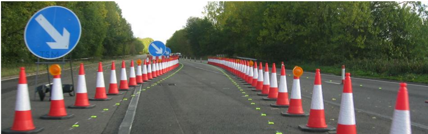
Typical traffic management arrangement for lane narrowing
