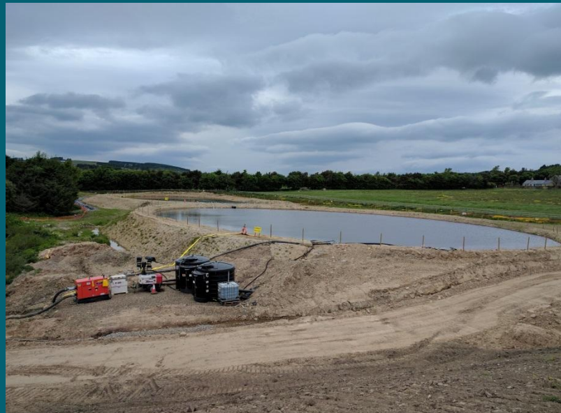
SuDS pond under construction
