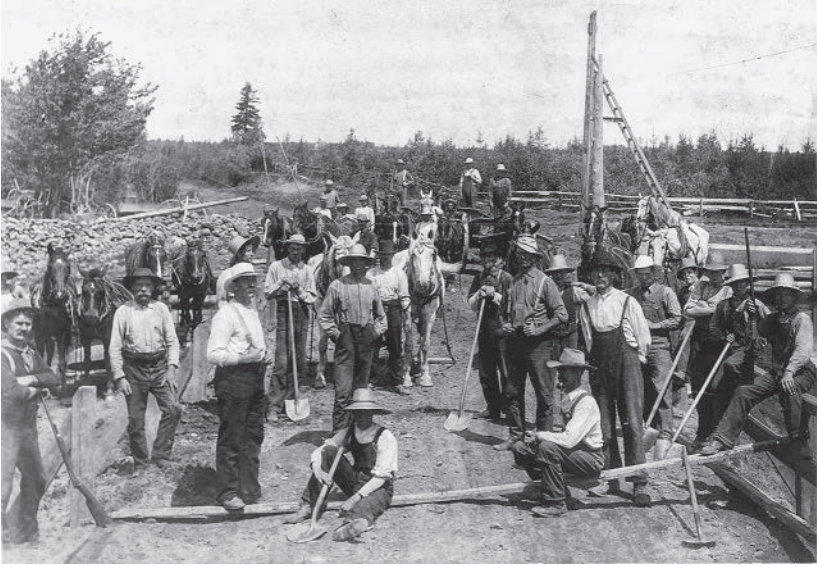
FIGURE 1.7 Work crew on the Wallace Bay aboiteau, ca. 1910. Courtesy North Cumberland Historical Society.
