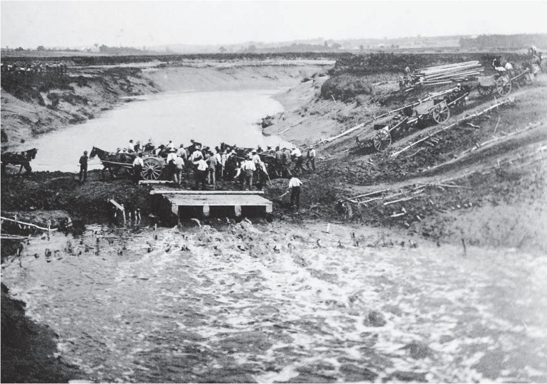
FIGURE 1.10 Repairing aboiteau after tiding, Falmouth Village Great Dyke Marsh Body, 1906. Courtesy Philip Davison, Falmouth, NS.
