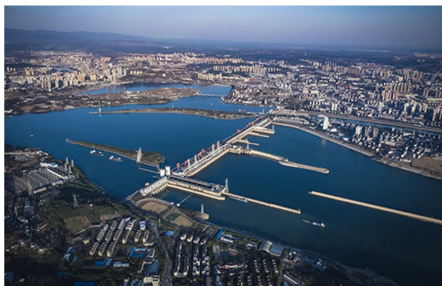
Figure 5. Gezhouba Dam, China.
