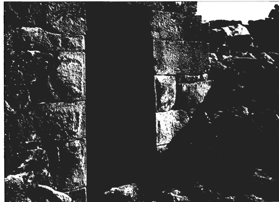
Photograph 3. Doorway in monastic complex at Umm es-Surab, Jordan, fifteen kilometres south of Bostra, possibly on the route Abu Talib's caravan might have taken. Though the location of Bahira's cell is not known, a room such as this would fit the conditions of the monk's residence much better than the Basilica in Bostra. Photograph by Bert de Vries
