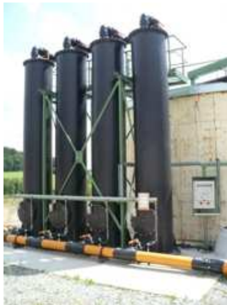
Abb. 24 H_2S - Biofilter
