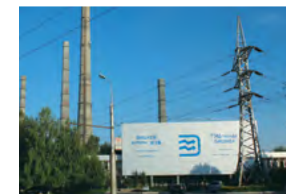
Bishkek Central Heating and Power Plant, © Grebnev V.V.
