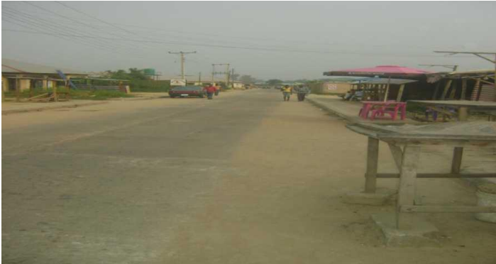
Fig 22: Agumagu Street, Yenagoa (one of the various streets that needed to be planted up)
