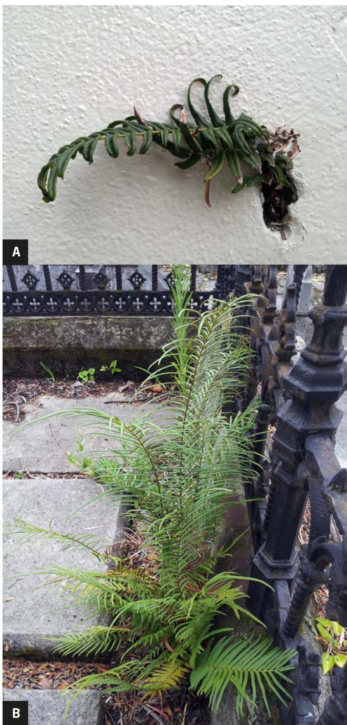
Figure 1. Pteris vittata : (A) young plant growing in mortar crack in painted-over concrete block/stucco external public toilet wall, Okahu Bay, Orakei Basin, Auckland, 14 June 2015; (B) mature plant growing amongst concrete slabs, Old Cemetery, Napier Botanic Gardens, Hospital Hill, Napier, 8 February 2016. Photographs © P. J. de Lange.
