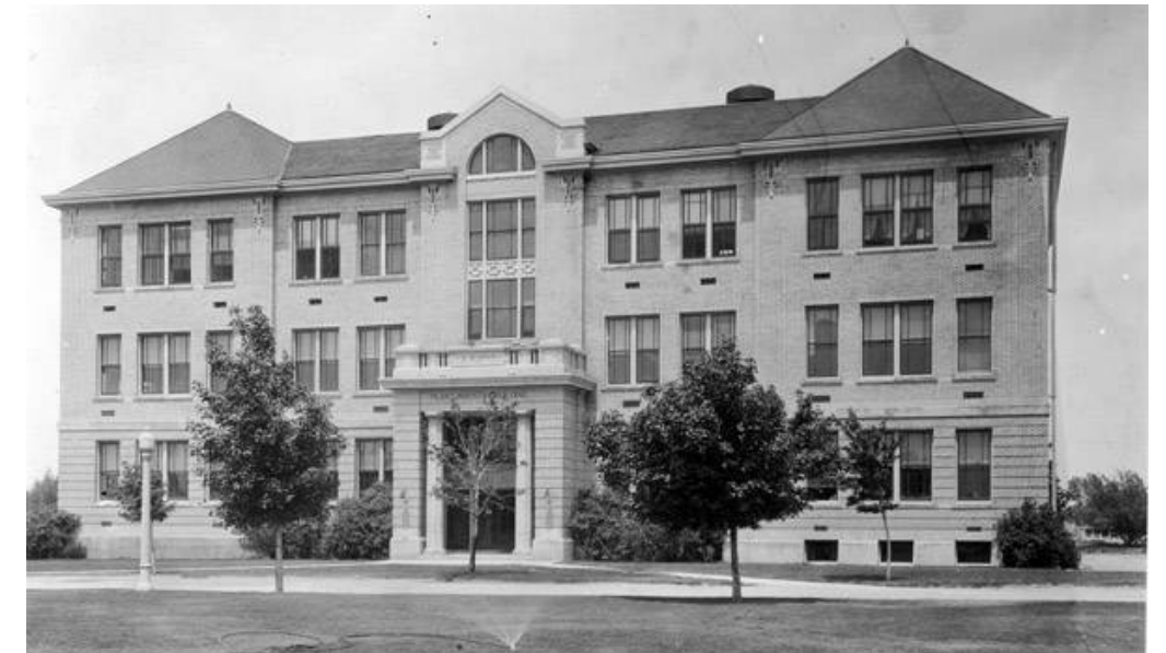
View of the Geology (Plant Industry) building, 1921
