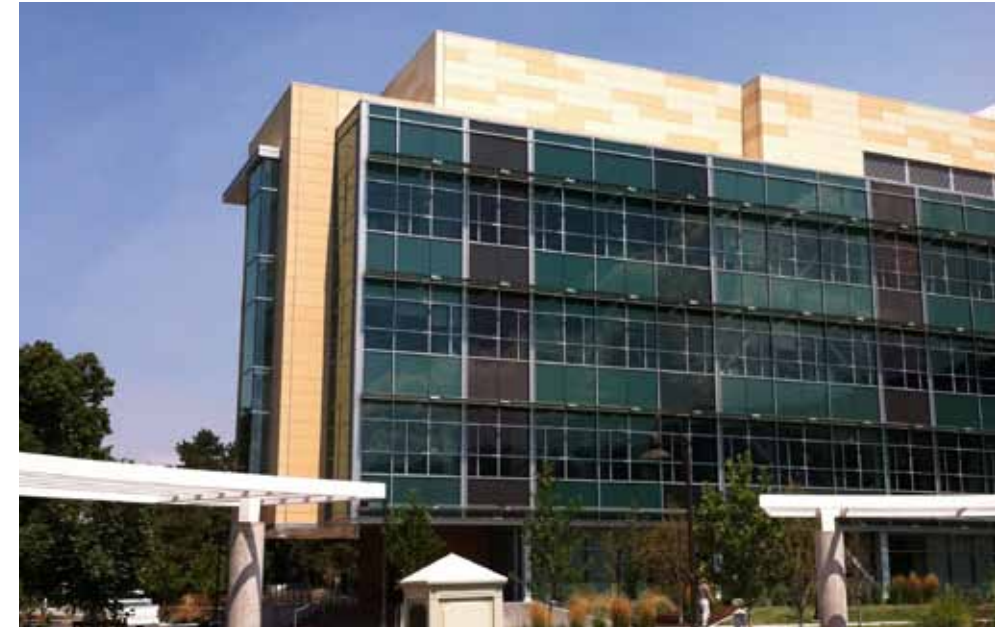
Building-integrated photovoltaics at the Agricultural Sciences building
