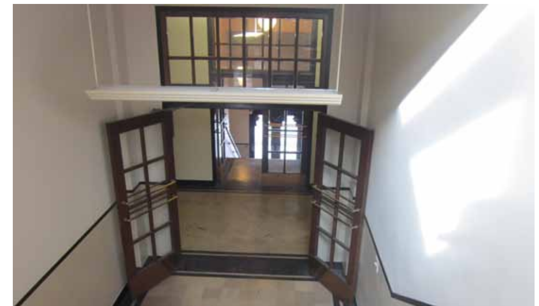
Stairwell, with original flooring, doors, and windows
