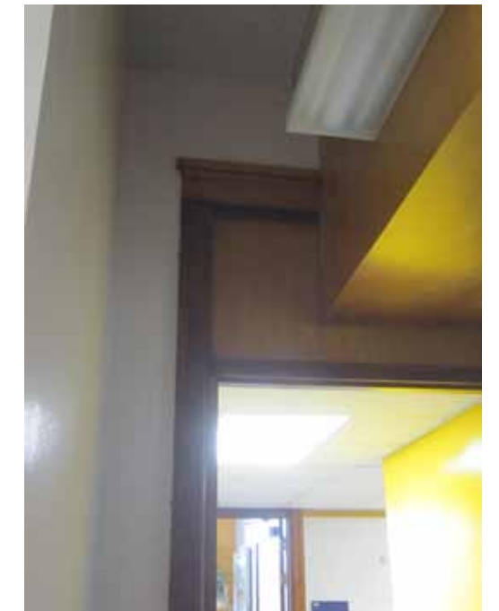
Dropped vs. original ceiling height
