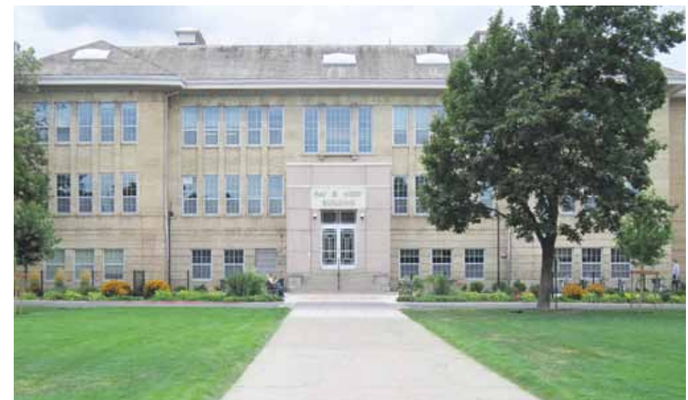
Retro-commissioning of existing facilities such as Ray B. West could identify potential options to maximize building system efficiency
