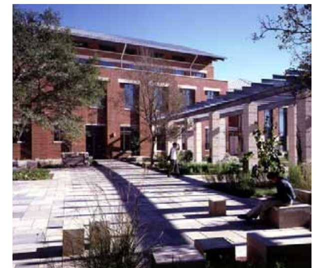
High albedo paving materials reflect the sun's rays to avoid creating heat energy
