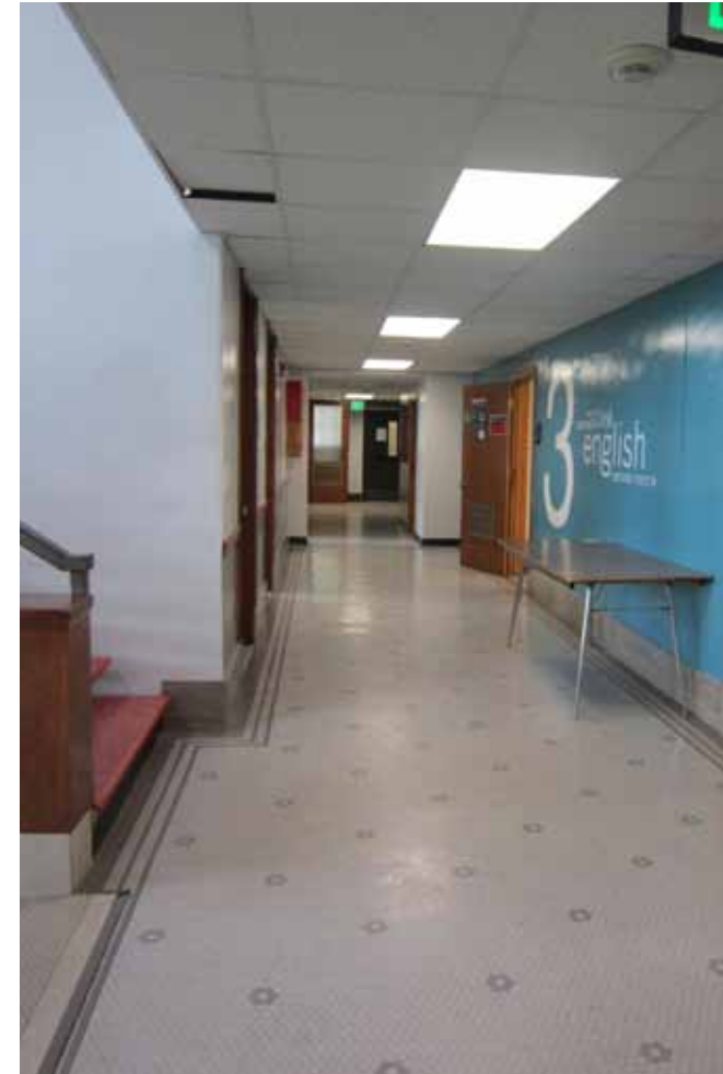
Existing facilities inside Ray B. West
