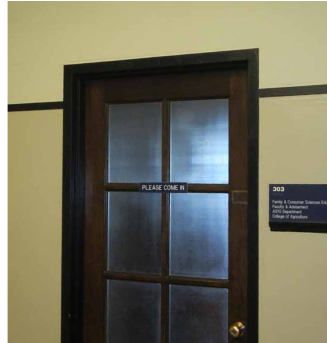
While offering original historic character to the interior of the Family Life Building, the function of the doors into public office space are limited by the opaque glass panes.
