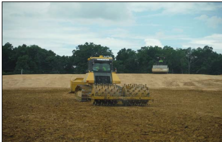
Figure C-31. Maxey Flats, KY Final Cover Construction in Progress (2015)
