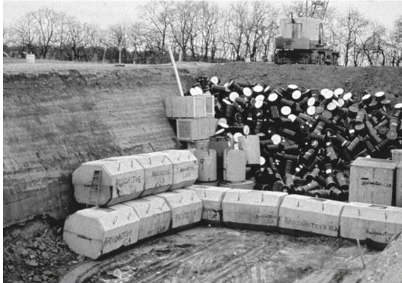
Figure C-35. Sheffield, IL Unlined Trench Burial of Waste during 1960s
