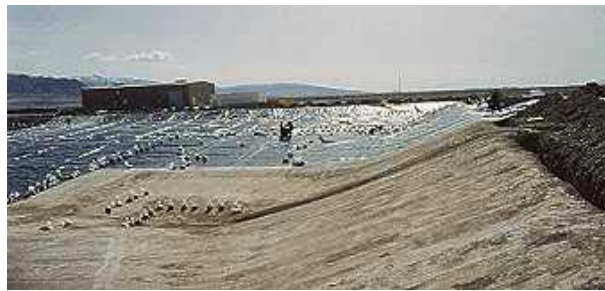
Figure C-5. Clive, UT Mixed Waste Liner Placement
