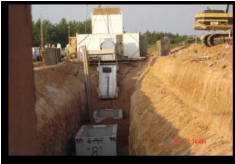
Figure C-15. Barnwell, SC Concrete Vault Placement
