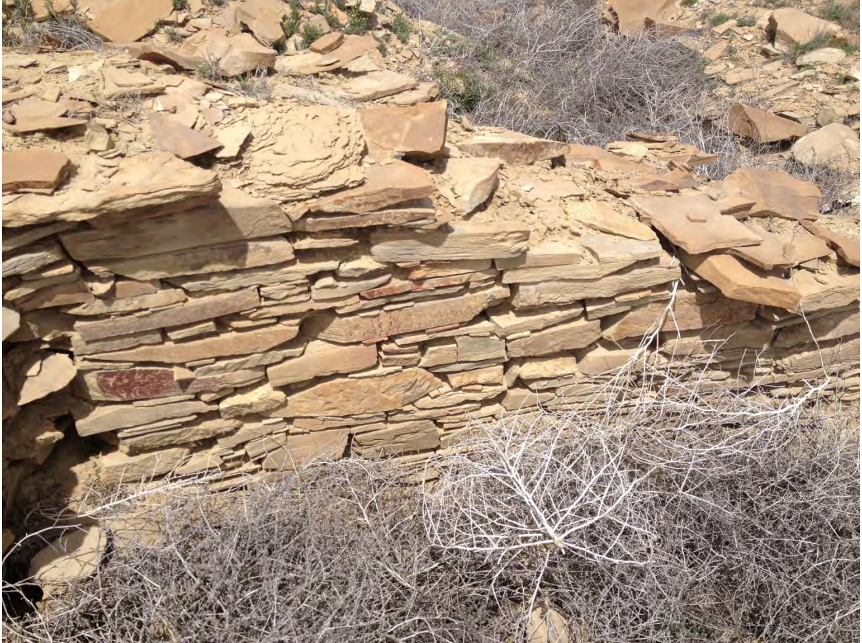
Figure 2.8. Exposed “Type II” Chacoan wall at Ruins Corner (LA 2520).
