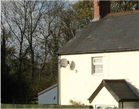
Highly visible satellite dishes can detract from the character of the Conservation Area.
