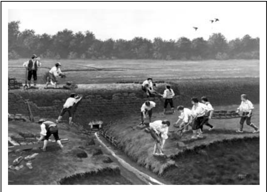
Figure 2. Acadians repairing a dike ( aboiteau ), c. 1720. Re-creation by Azor Vienneau. Source: Nova Scotia Museum, N-12,212.
