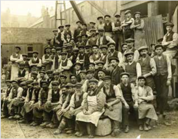
Workmen at Victoria Road Granite Works
