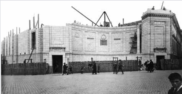
Cowdray Hall/War Memorial under construction, circa 1924
