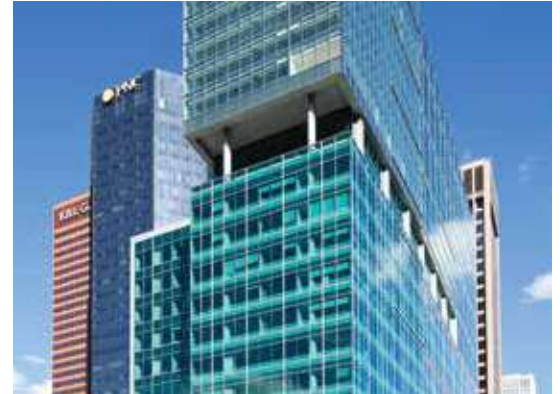
Three PNC Plaza | Pittsburgh, Pennsylvania - EE.UU. | Arquitecto: Gensler | Procesador Certificado Vitro: Trulite Glass and Aluminum Solutions | Instalador: Oldcastle BuildingEnvelope
