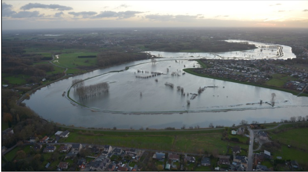
Figure 2 FCA/CRT 'Bergenmeersen' filled during storm surge of 6 th of December 2013 (© Hydrologic Information Centre, Flanders Hydraulics)
