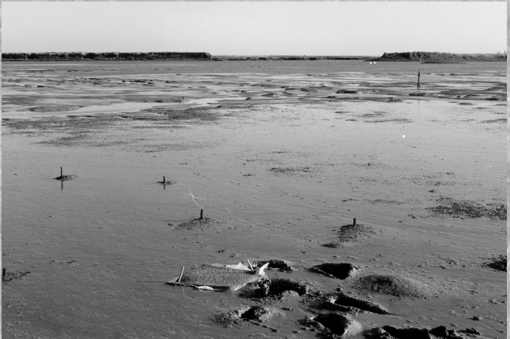
Astroturf mat at Tollesbury with the breach in the embankment at the horizon
