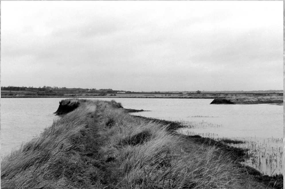
De-embankment at Tollesbury
