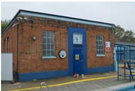
Figure 4.25: Pump Room, northern elevation.
