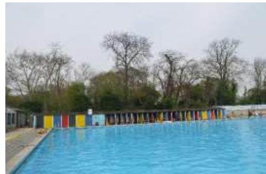
Figure 4.20: Changing rooms to the western side of the pool.
