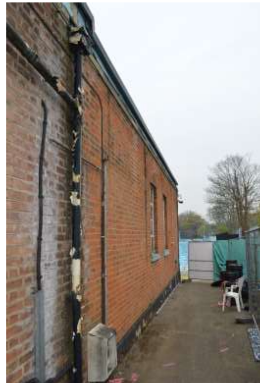
Figure 4.30: Pump Room's (Northern Building) eastern elevation.
