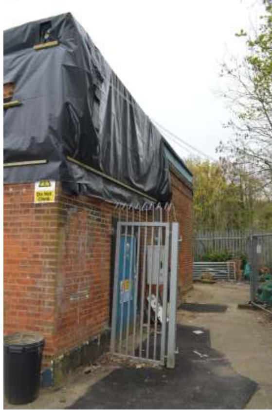
Figure 4.31: Southern elevation of the Pump Room's Southern Building.
