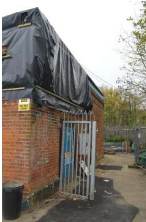
Figure 6.20: Southern Elevation of Southern Building.
