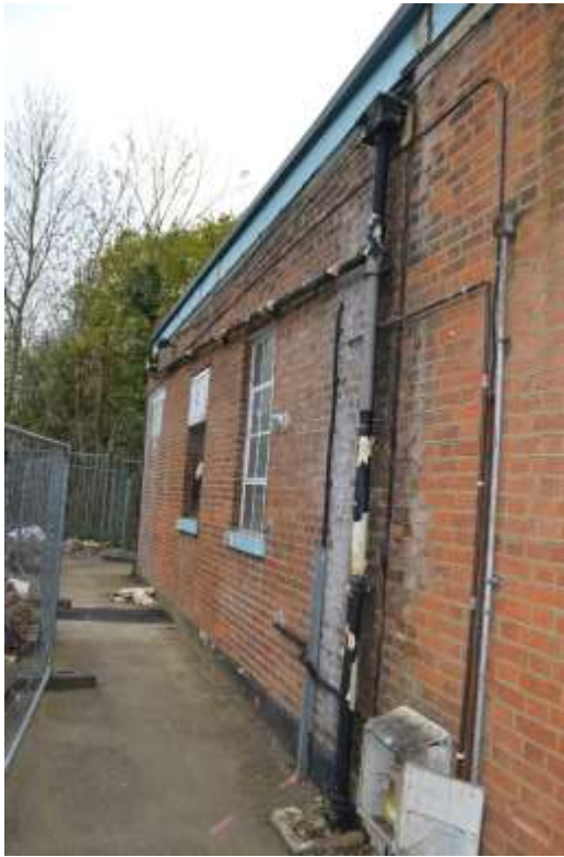
Figure 4.29: Pump Room's (Southern Building) eastern elevation.
