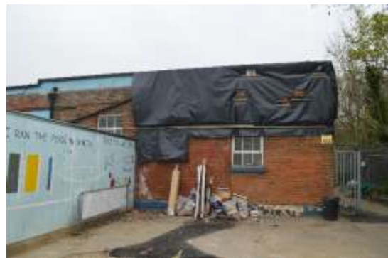
Figure 4.26: Pump Room's (Southern Building) western elevation, south-western corner.
