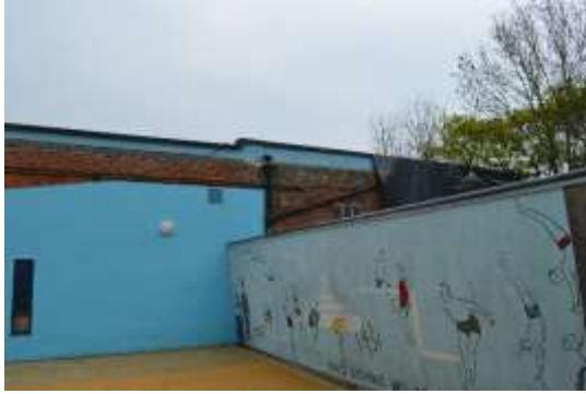
Figure 4.27: Pump Room, western elevation. Note part cordoned off.
