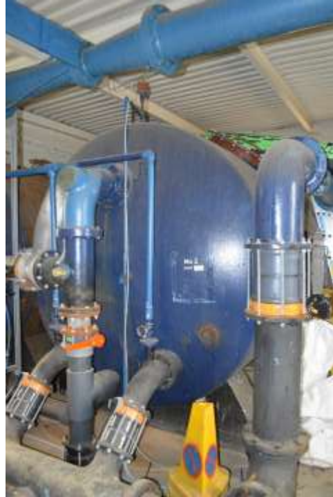
Figure 6.22: One of the cylinders to the Southern Building.
