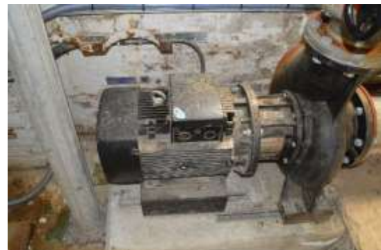
Figure 6.30: Modern plant in the north-western corner.
