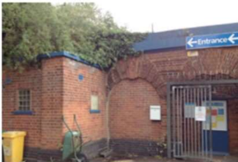
Figure 4.13: The entrance arches prior to demolition, southern elevation.
