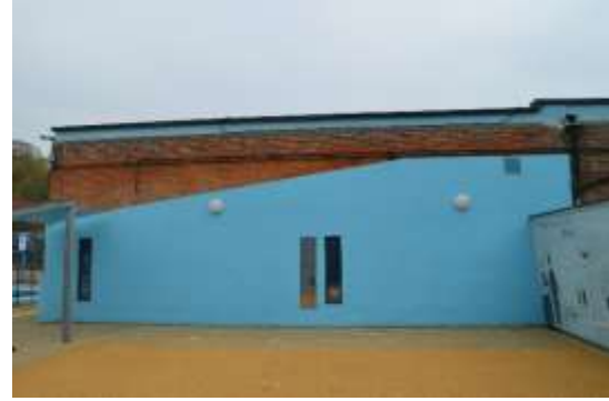
Figure 4.28: Pump Room's (Northern Building) western elevation.
