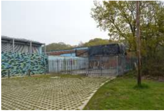
Figure 4.15: South-western corner of the Pump Room adjoining the new pavilion.
