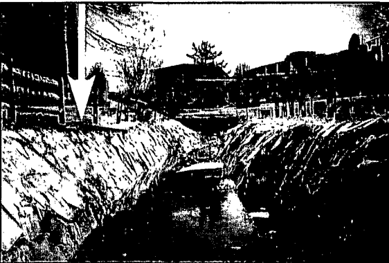
Poor Range (MD Save Our Streams) (arrow pointing to channelized streambank with no vegetative cover)
