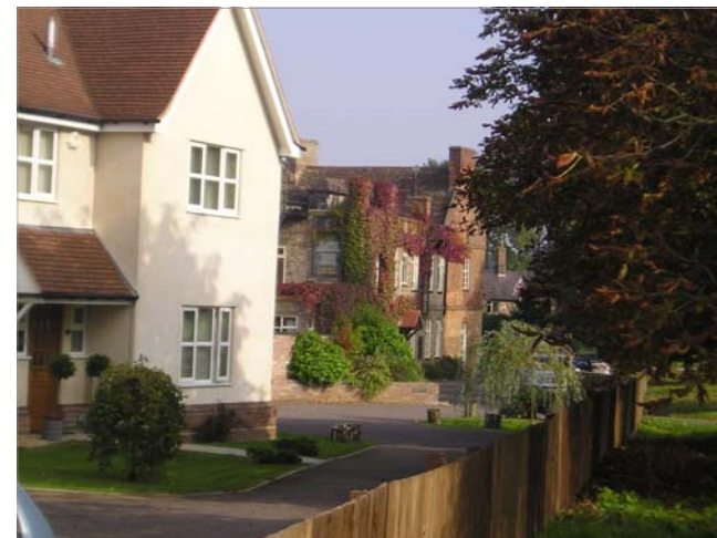
Fig 3. Newly built houses in Chestnut Close and The Olde Bull in successful visual harmony
