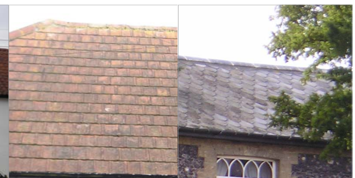
Fig 41 Flat interlocking clay tiles. Tiles made from the local gault clay are pale pink and pale yellow. Plain or peg
