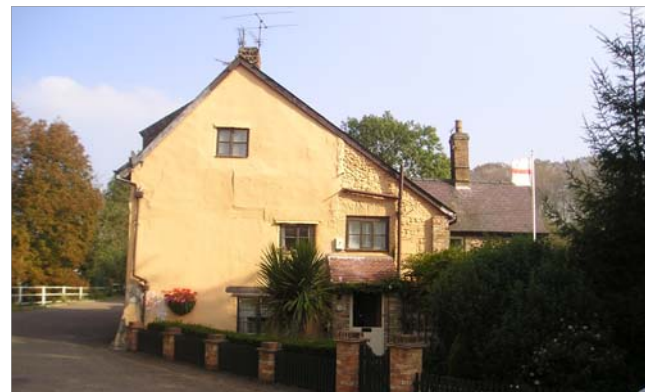
Fig 48, Larkspur Cottage: Painted lime-render on timber-frame
