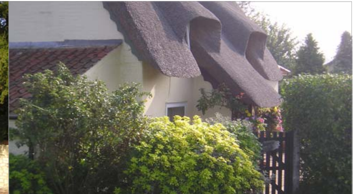
Fig 39, Eyebrow dormers in reed thatch
