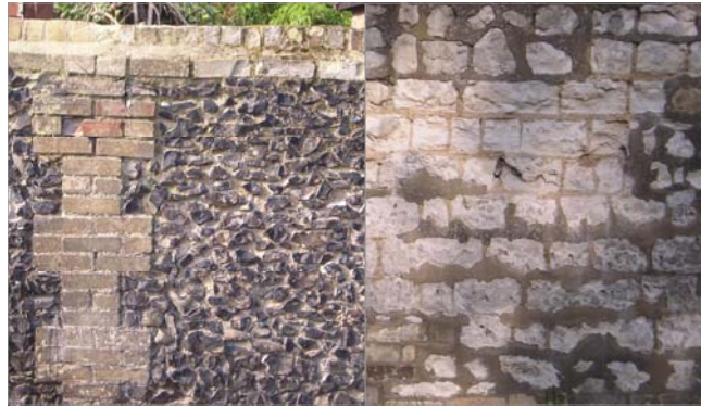
44, Napped flint & gault brick Fig 46, Chalk block or clunch
