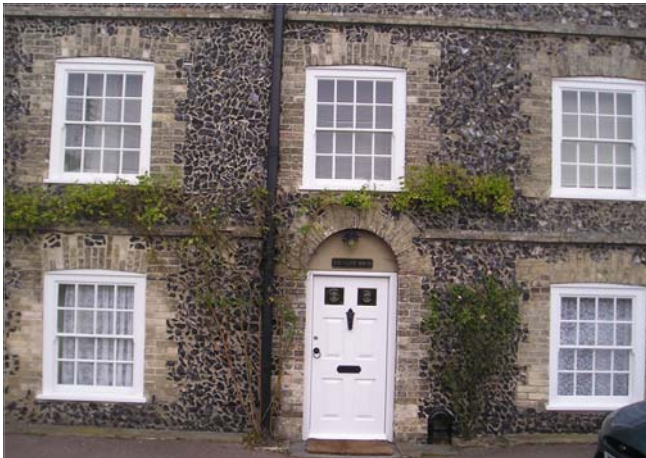
Fig 31, The napped flint and gault brick Classical Façade of No.1 Church Lane
