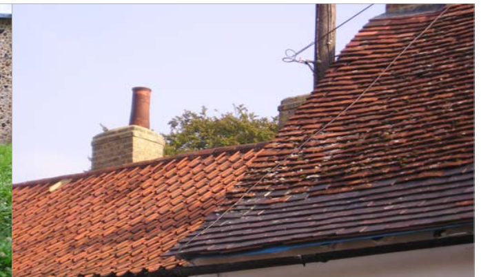
Fig 40, Red clay pantiles to left; hand made plain tiles above right & machine made plain tiles below right.
