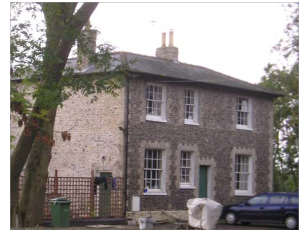
Fig 26, Poplar Villa undergoing restoration.
