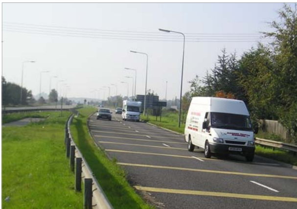
Fig 12, The A11 trunk road as it passes close to the village
