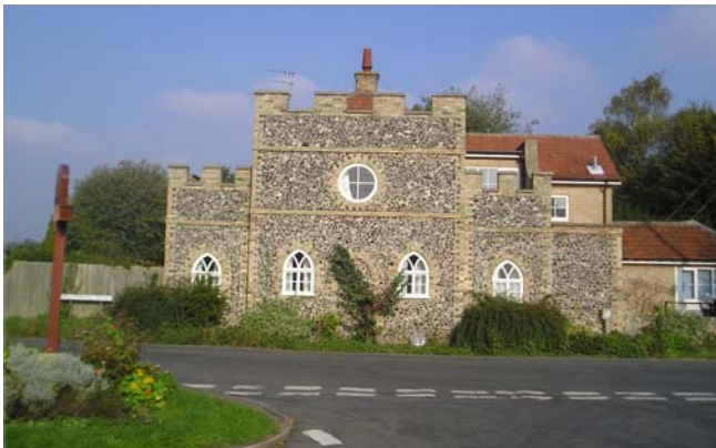
Fig 32 Glebe Cottage, No 1 The Street a rare Georgian gothic facade
