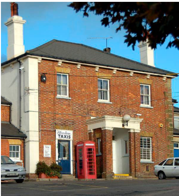
Fig. 6. The railway station (1858).
