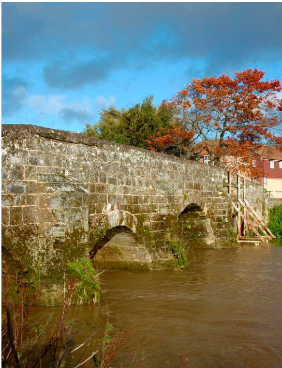
Fig. 4. Pulborough bridge (1785) from the south-east.
