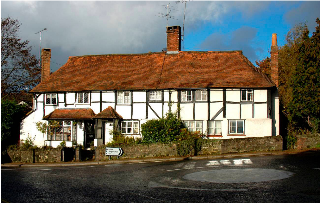
Fig. 11. Swan Cottage, Horncroft and Old Timbers, Church Hill: 16 th -century timber framing.
