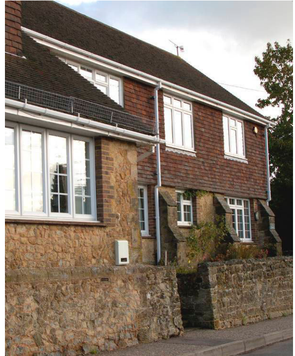
Fig. 7. The school (1857), closed 1972 and converted to residential use.
