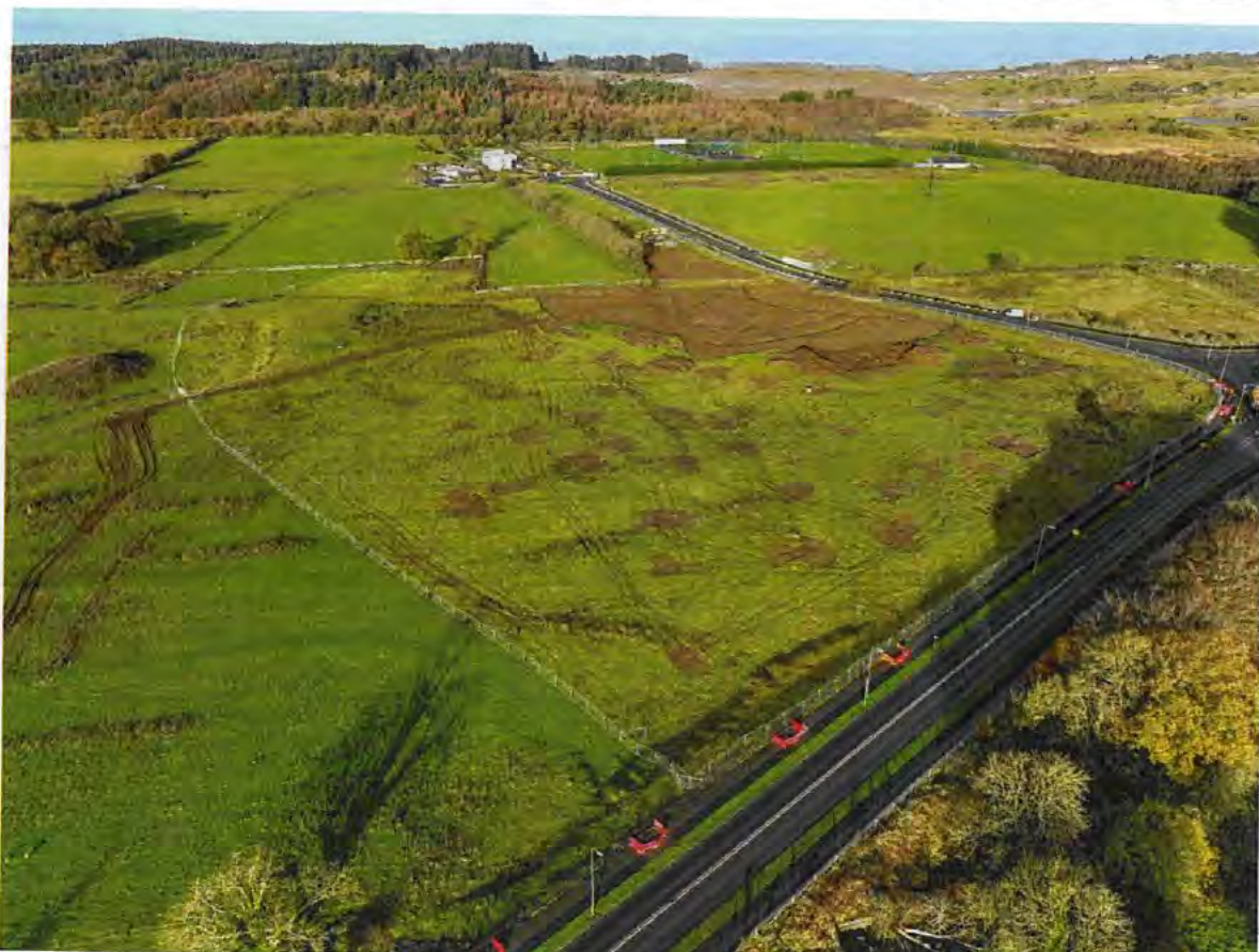
Plate 1: Aerial Image of Lands
