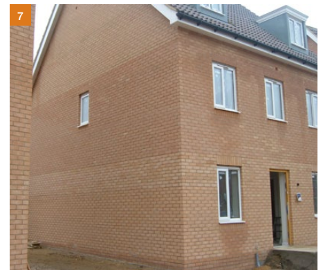
BELOW: Poor blending of bricks can result in unsightly banding or demarcation lines.
