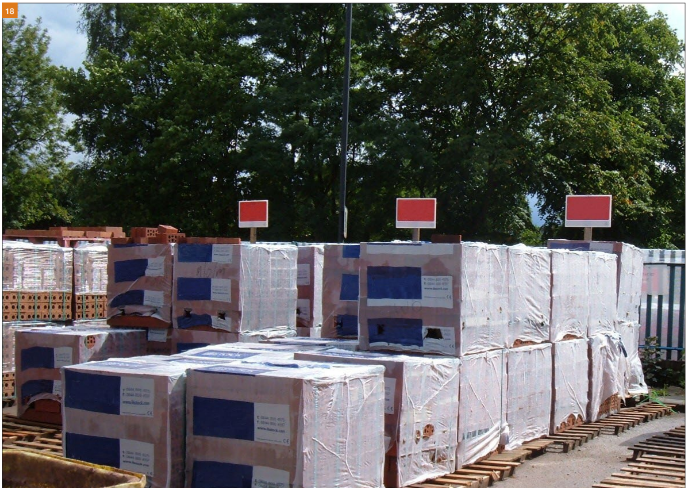
Well marked brick bays.
