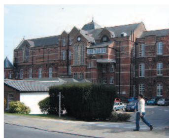
Royal Hampshire County Hospital
