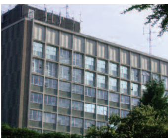
Hampshire Police Headquarters
