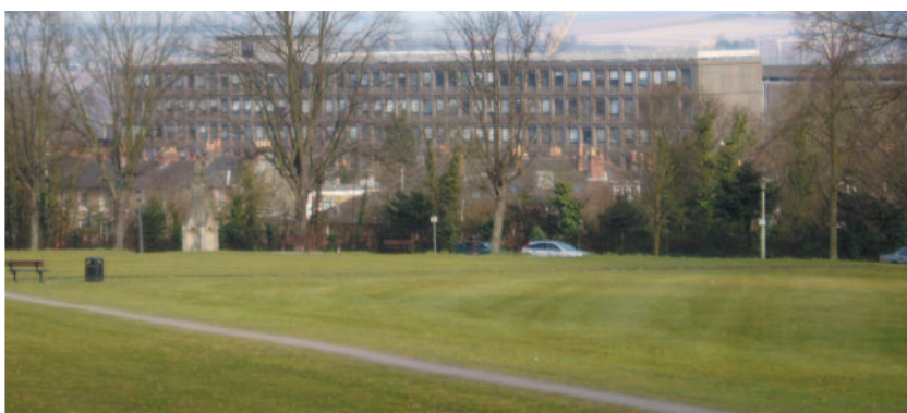
Ashburton Court before refurbishment seen across the Arbour
