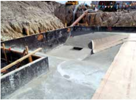
Figure 10. A horizontal bentonite waterproofing sheet being placed at the elevator pit.
