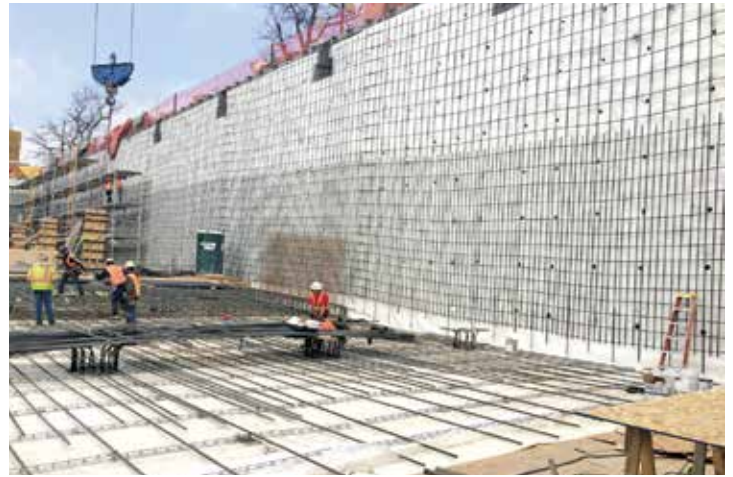
Figure 14. Reinforcing steel being installed over the top of preapplied sheet waterproofing.
