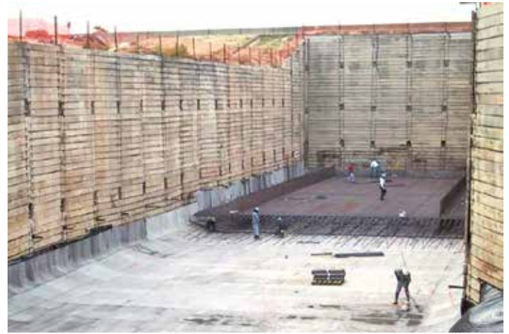
Figure 4. Mat slab under construction.
