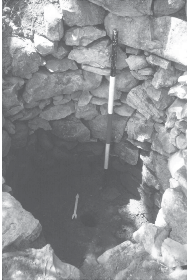
Figure 37. Site 44AU634, Feature 12, north view.
