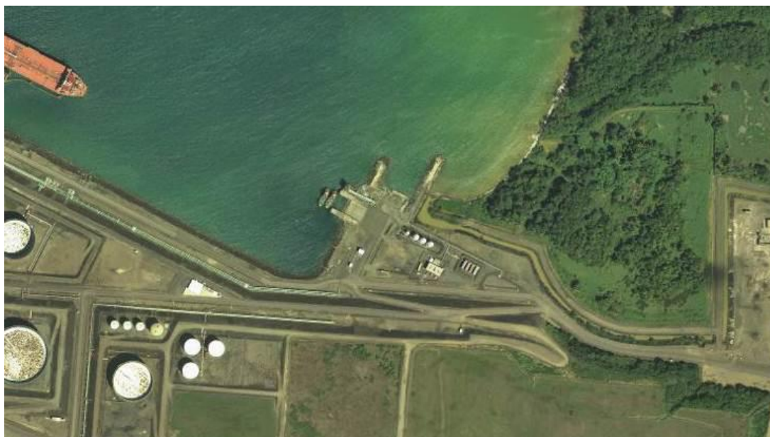
Figure 3.6 Aerial photo of Hess Oil Terminal in Cul de Sac, Source: The Physical Planning Section, tile 0645.
